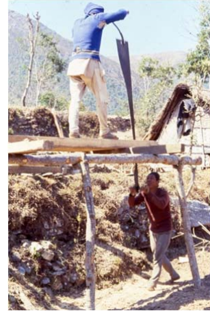
Rebuilding following the earthquake, 1988
