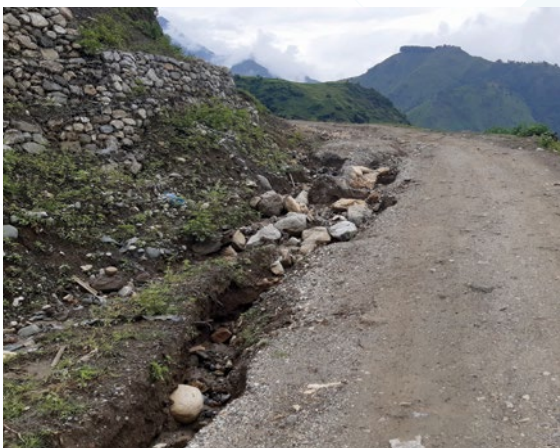
Unmanaged roadside drainage canal increasing road accident and landslide risks.
