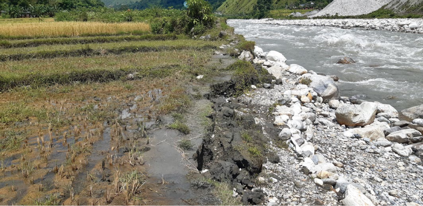
Soil erosion due to haphazard rock and sand excavation.
