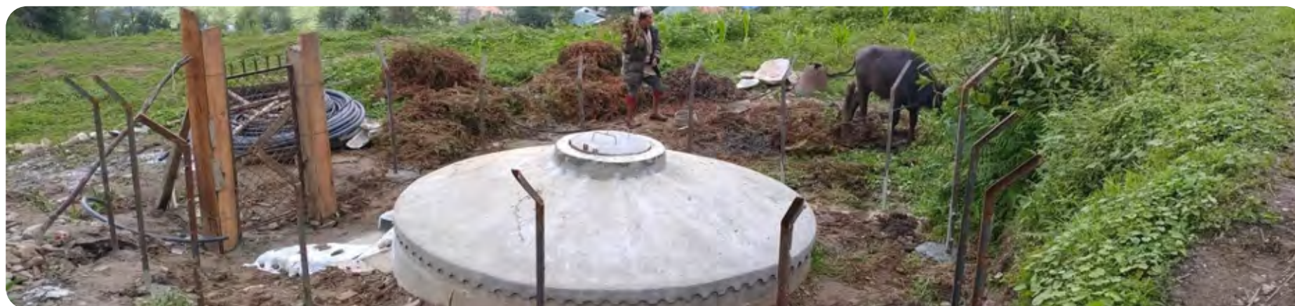
Reservoir tank of Thading Water Supply Scheme under construction at Tipling.
