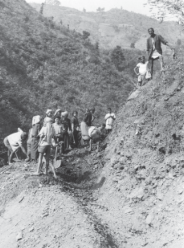
Work on irrigation canals, Nawal Parasi
