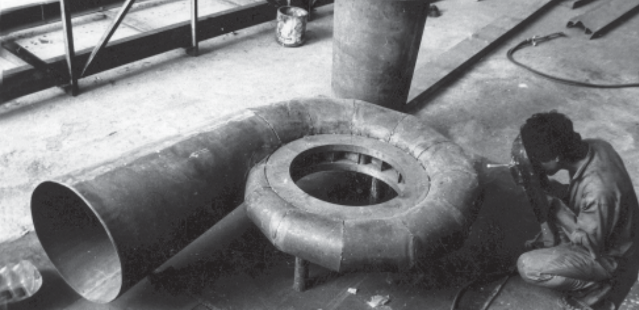
Turbine casting at Nepal Hydro Electric
