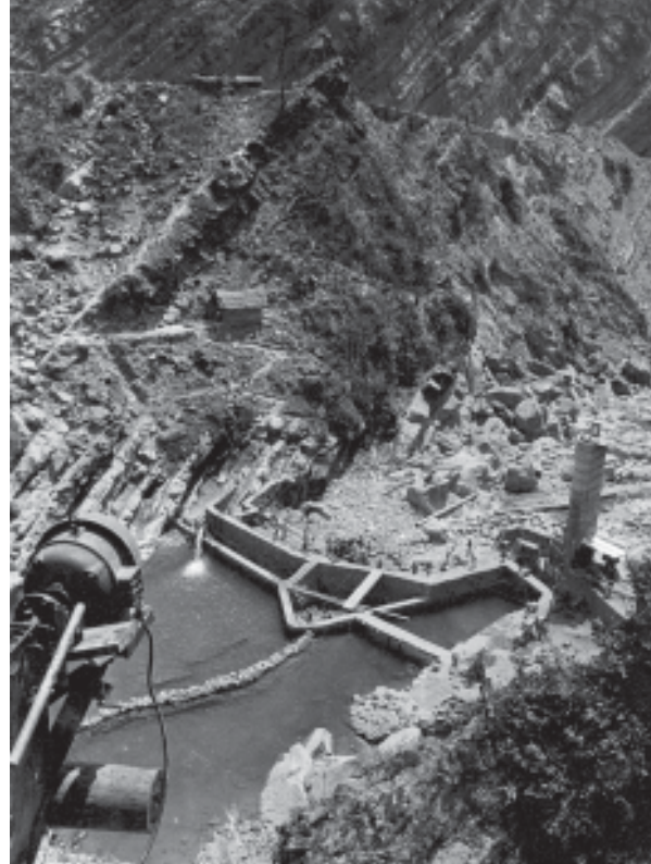
Tinau dam completed in 1977-78
